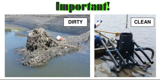
Recently, the NEW aerators at the wastewater treatment plant weren't functioning properly. After attempting various remedies, the manufacturer of the aerators came to inspect the equipment. They immediately found the reason that the aerators were not working. It was due to over **twenty five pounds of rags and paper-type material on just ONE of the 24 aerators in the ponds!**
