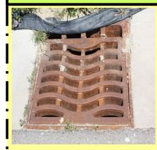
Storm drains are an important feature within your community because during heavy rainstorms, the drains reduce flooding in streets and neighborhoods by transporting large volumes of water into rivers quickly. Filters are not installed in the drains because they would delay the passage of water. Therefore, whatever goes down storm drains will end up in your waterways (rivers, streams, lakes, creeks and oceans).
